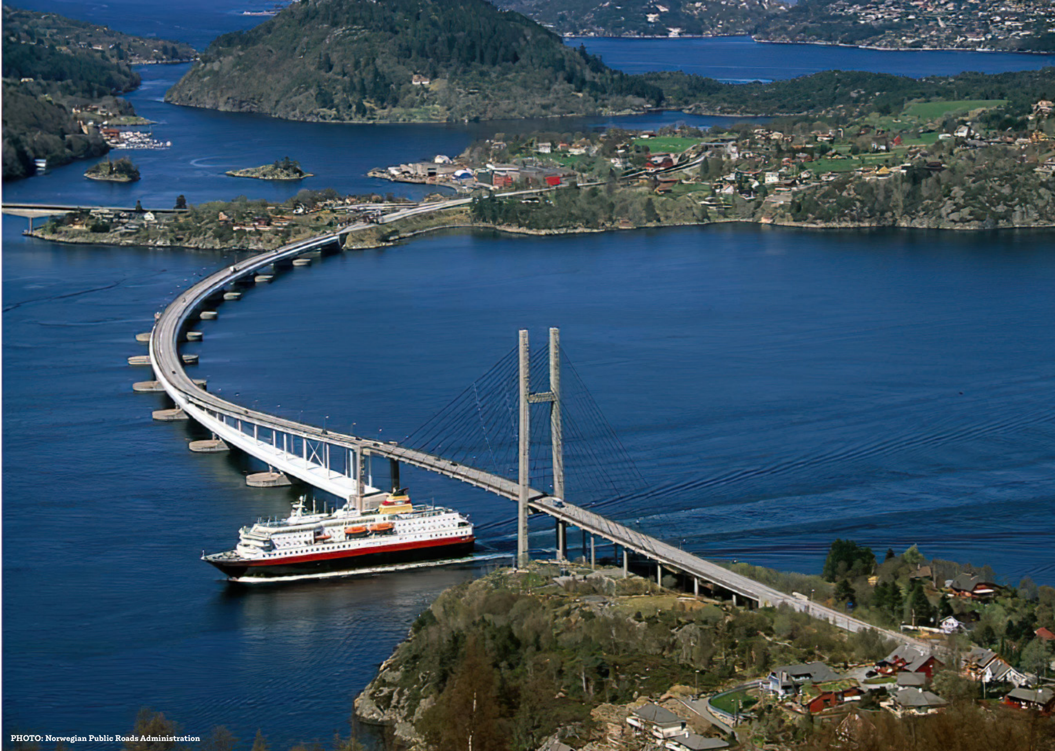
Nordland Bridge in Norway was built with pontoons perpendicular to the road deck, allowing for greater fish passage.
