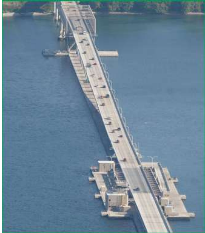
Figure 33. Light luminaries on the east half of the Hood Canal Bridge. Image courtesy WSDOT.
