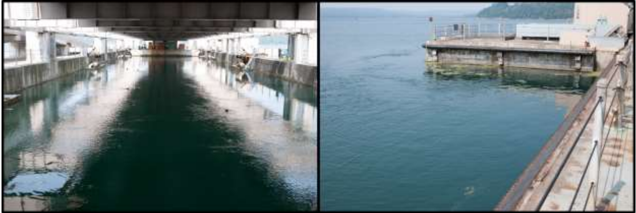
Figure 3. On left, the east bridge pool area, looking towards the closed center drawspan. On right, one of the corner areas created by cross-pontoons that jut out from the bridge structure. Photos courtesy of LLTK.
