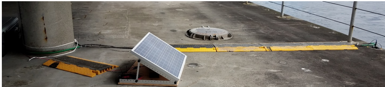
Figure 2.4: Routing of sensor cables and position of solar panel
