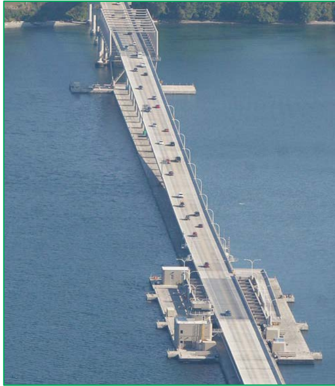
Figure 2-4. Light luminaries on the east half of the Hood Canal Bridge, Washington (adapted from Rodda 2020).
