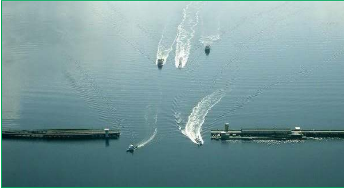
Figure 2-3. Scheduled fish passage bridge opening on Hood Canal Bridge, Washington (adapted from Rodda 2020).
