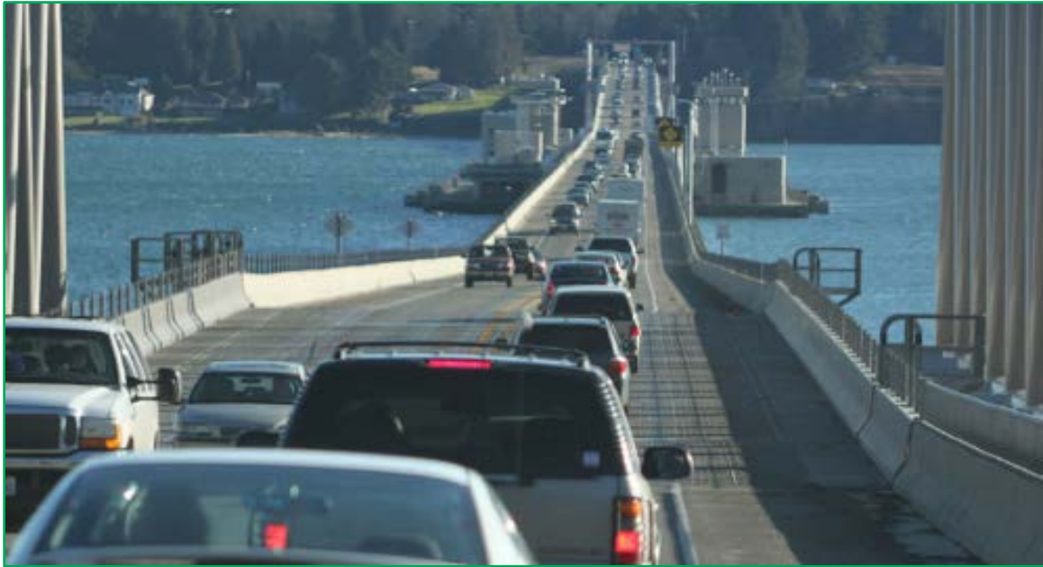
Figure 2-10. The number of cars passing Hood Canal Bridge, Washington approaches 15,000 on weekdays and 19,000 on weekends.
