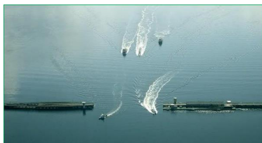
Figure 33. Vessels passing through the open Hood Canal Bridge drawspan. Image courtesy WSDOT.
